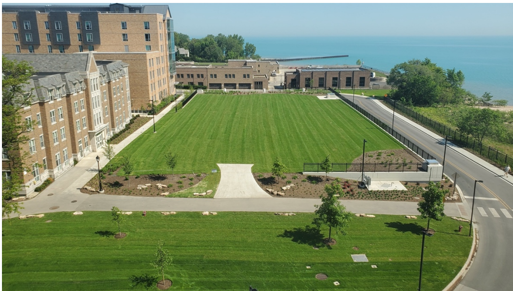
Above: Clearwell 9 Replacement Project post-construction
