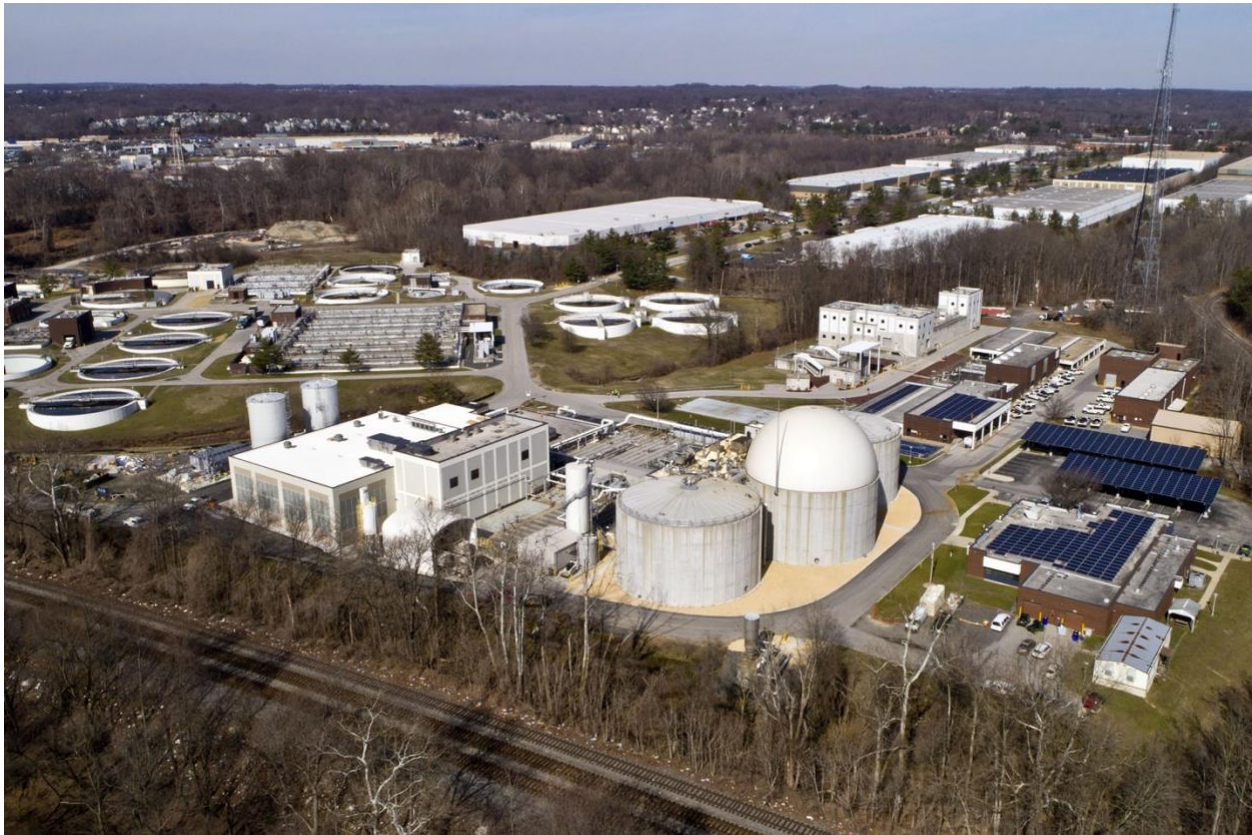
Howard County Little Patuxent Water Reclamation Plant (PWRP)
