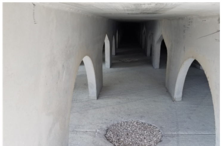
Albion Riverside Park (Four Photos Above)
